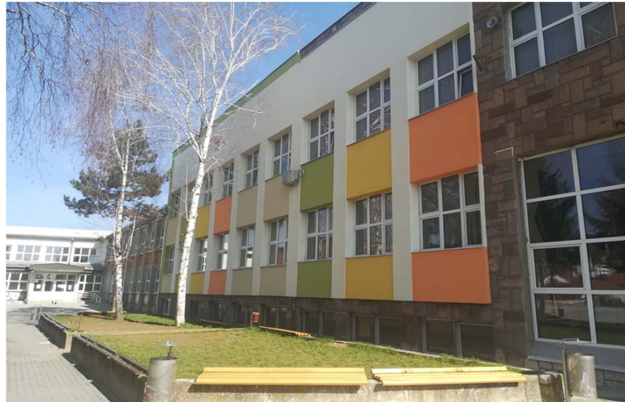
Primary School in Pirot
