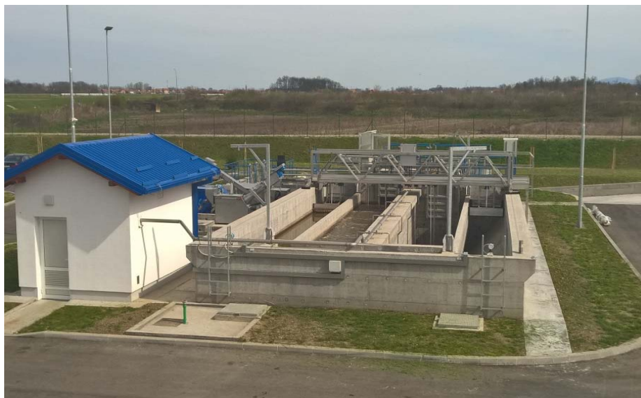
WWTP Site in Bijeljina
