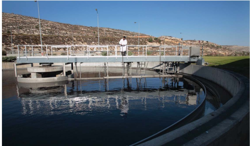
Wastewater Treatment Plant - secondary sedimentation
