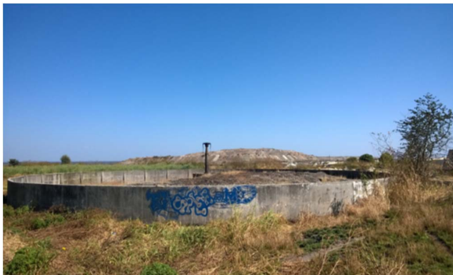
Copperbelt Province – Chingola – Old Trickling Filter at Ponds Site
