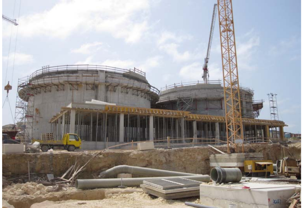
Digesters under Construction
