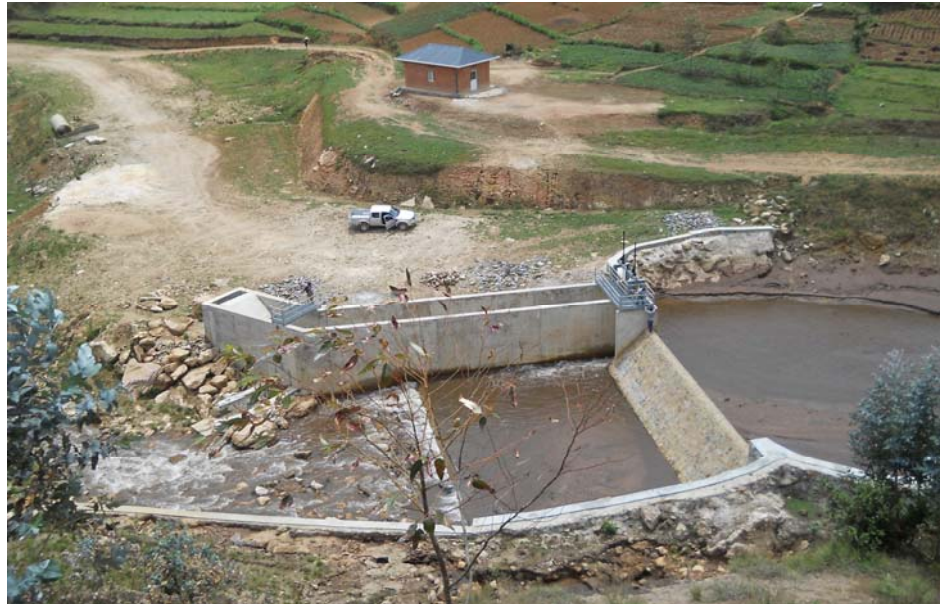
Template of an Intake Structure
