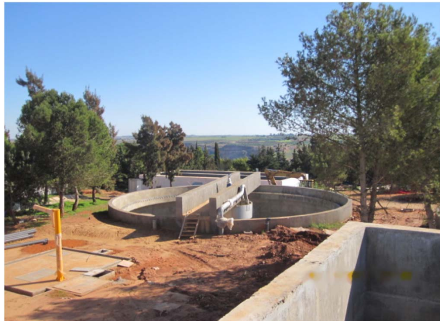
New Clarifier under construction, treatment plant Bouregreg
