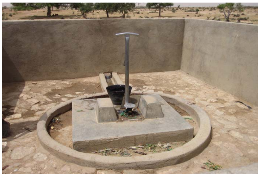
Drink water point with foot pump
